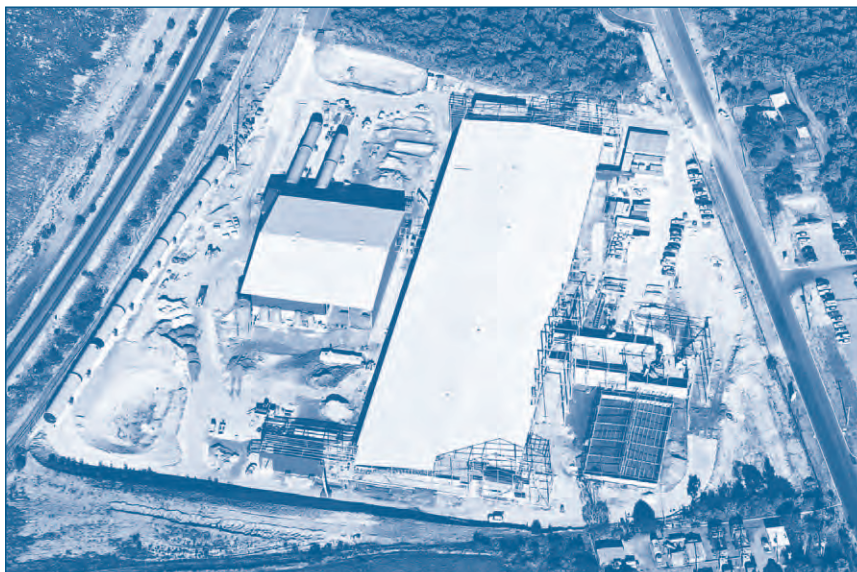
Construction of In-Vessel Composter, Regional Resource Recovery Centre (RRRC) Canning Vale
